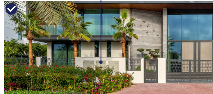
Non-compliant screening /Integration of Utility meters
