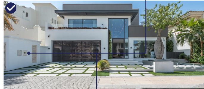
Screened / Integration of Wall Utility Meters
