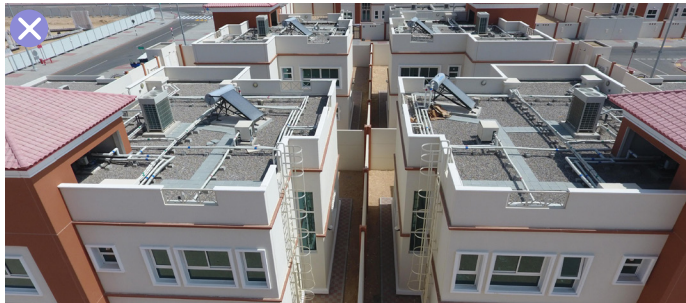
Non-compliant screening of MEP equipment
