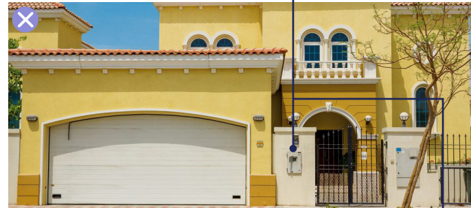
Non-compliant screening /Integration of Utility meters
