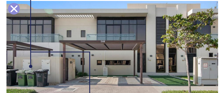
Non-compliant screening of Utility/Waste Room
