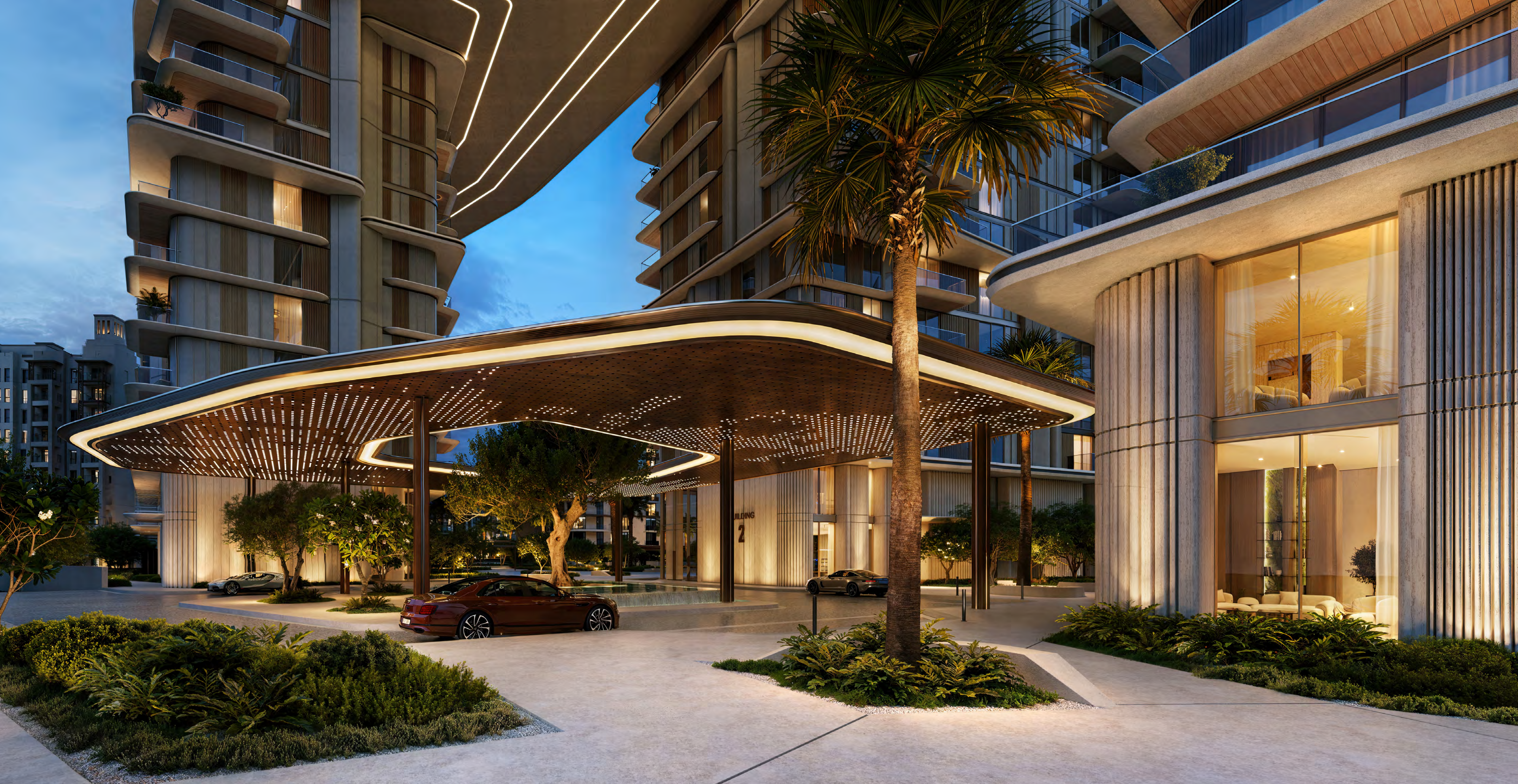
The drop-off area, set between the buildings and enhanced by greenery and a tranquil water feature, ensures convenient access while serving as a striking focal point of architectural elegance and natural beauty.
